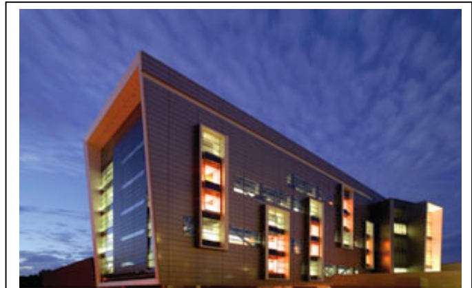
Headquarters of UCSD Division of Cal. Institute for Telecommunications and Information Technology (Calit2). Photo by Philipp Rittermann
